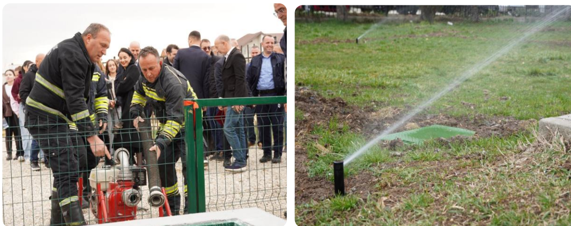
Photo 3: Testing the fire extinguisher and sprinkler system
